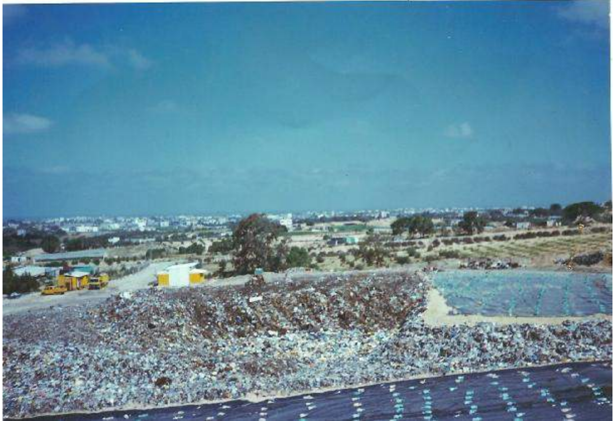
Photo (4) Plastic cover of the Dear Balah Landfill.
