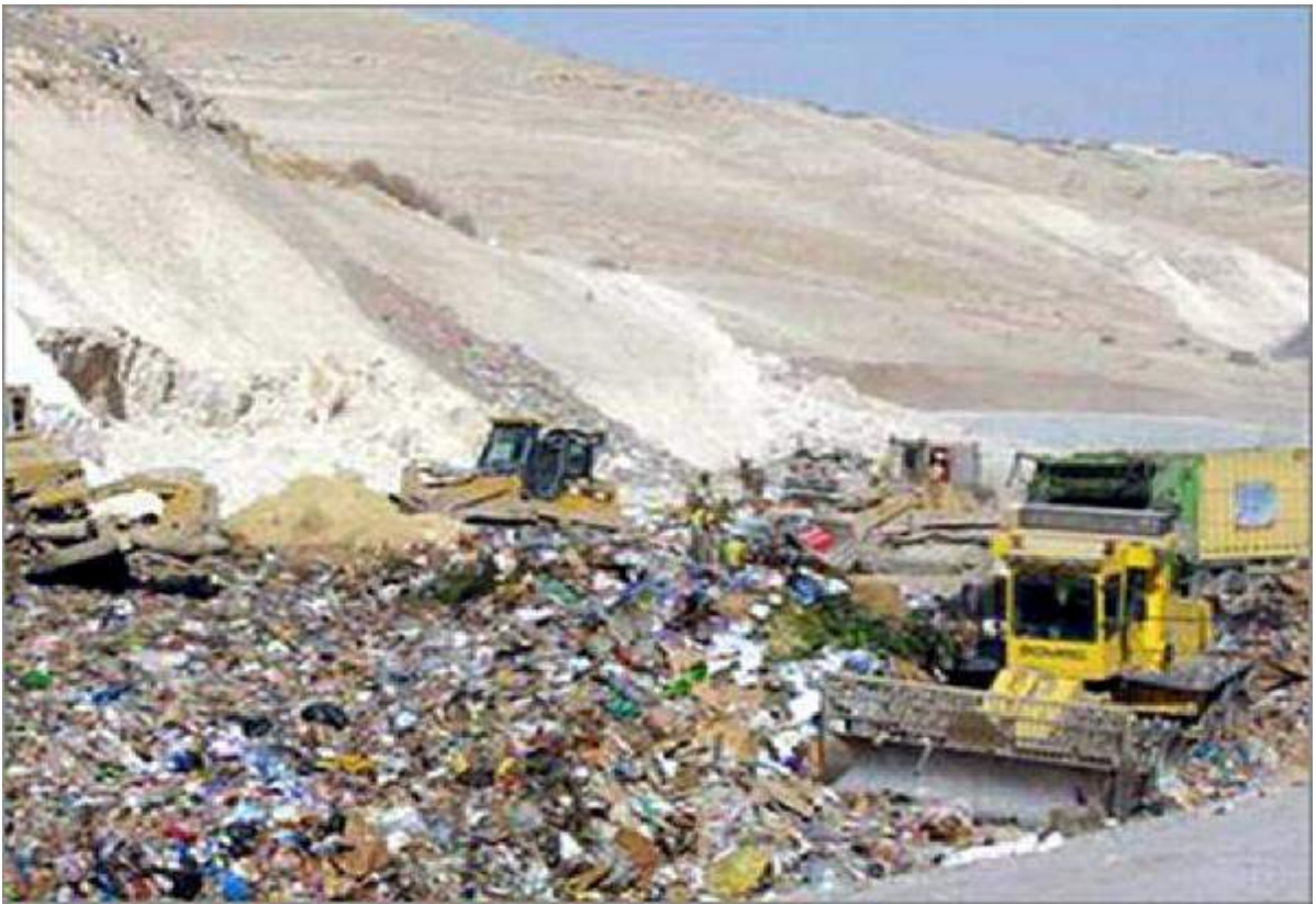
Photo (5) Soil cover of the Dear Balah Landfill
