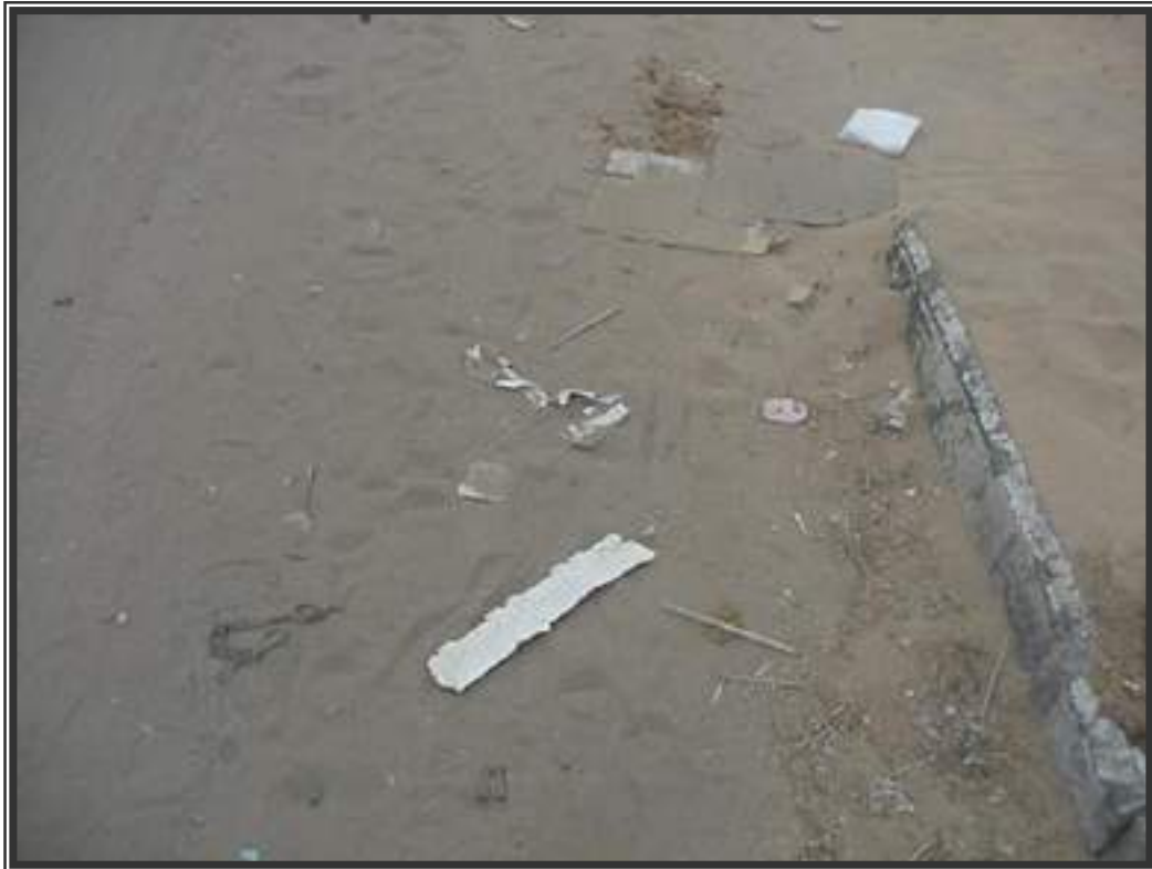
Fig. (2.4) Surface sediment of sand on the road near the gutter.
